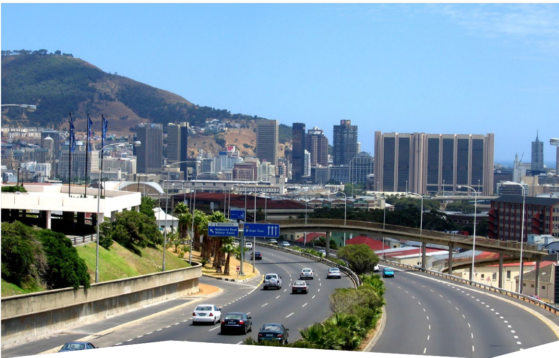
Sea Point Highway Cape Town, South Africa
