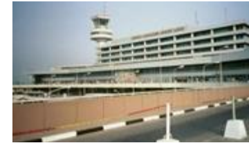
Nigeria Airport ISP, Africa
